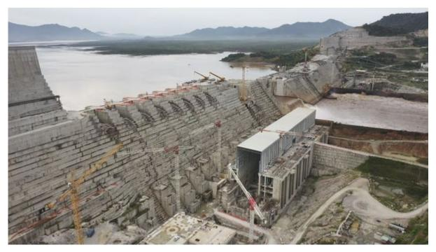
Aerial view of the Grand Ethiopian Renaissance Dam, during construction in late 2019. The turbines will sit at the bottom of the building. Water will enter a total of 16 turbines through the two round holes in the bottom of the wall, which will generate electricity for Ethiopians.EDWARD BURTYNSKY / COURTESY NICHOLAS METIVIER GALLERY, TORONTO
